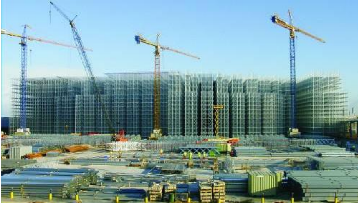
Quinn Glass Liverpool - 180 x 290 x 35 metres high 250,000 pallet capacity
